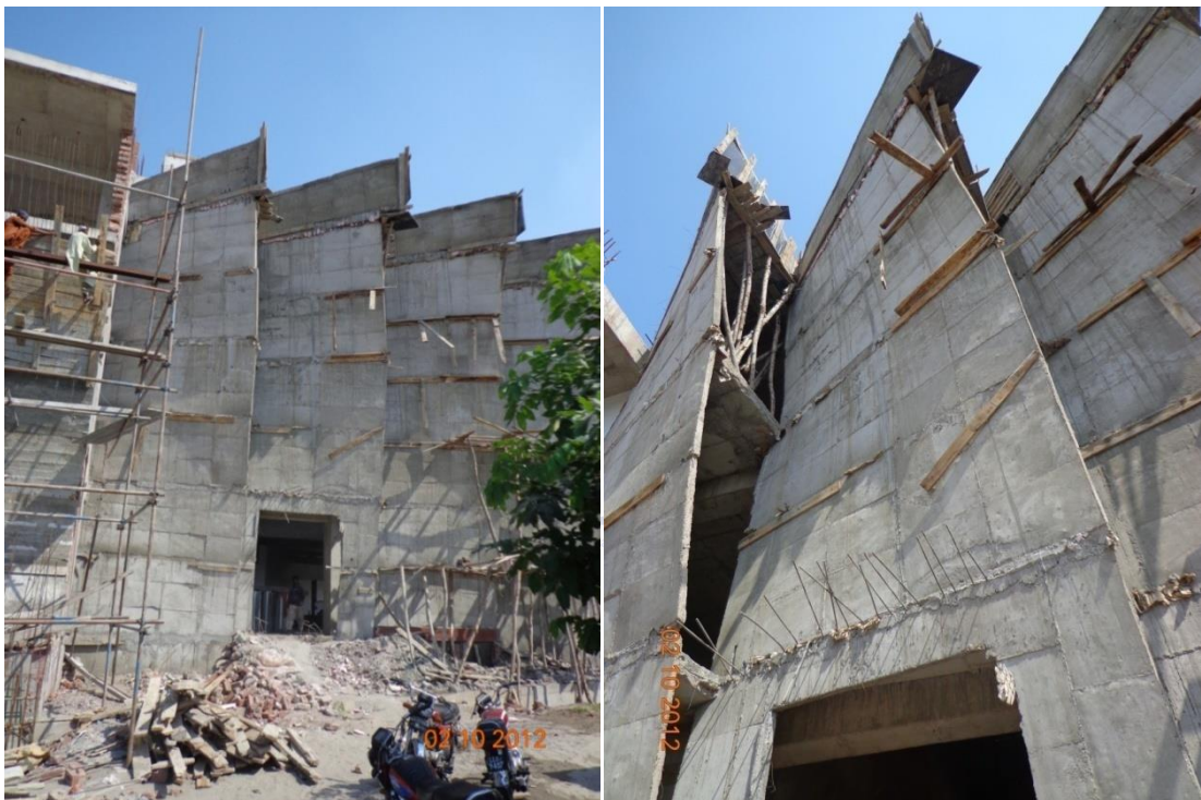
Fig 3 ,4 Main entrance to the club building
