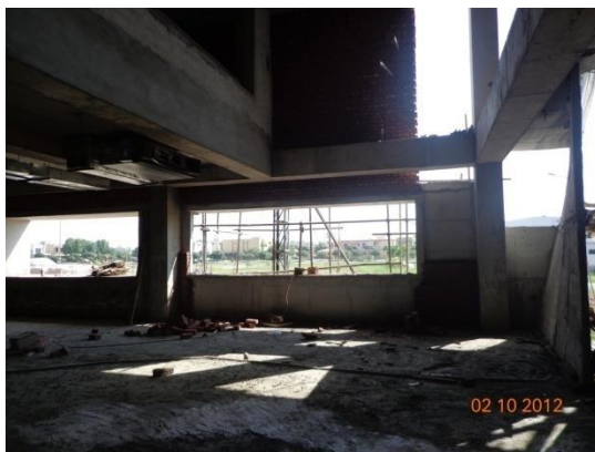
Fig 11 View of Entrance Lobby
