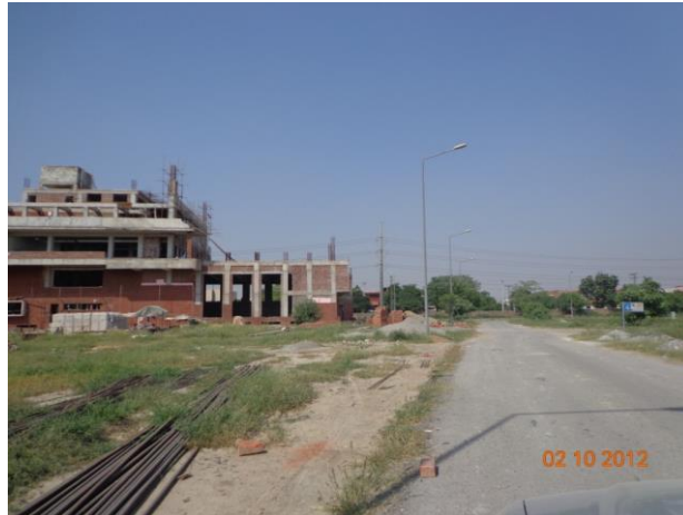
Fig 2 Access road to the site
