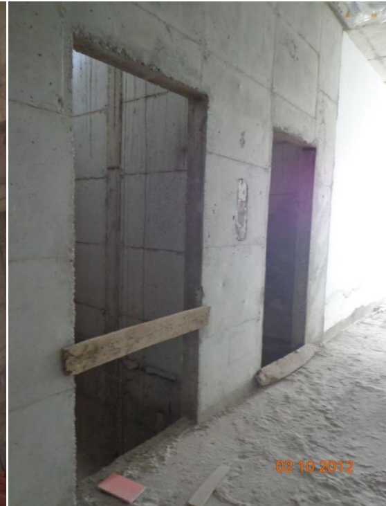
Fig-6 Lifts and Stair hall
