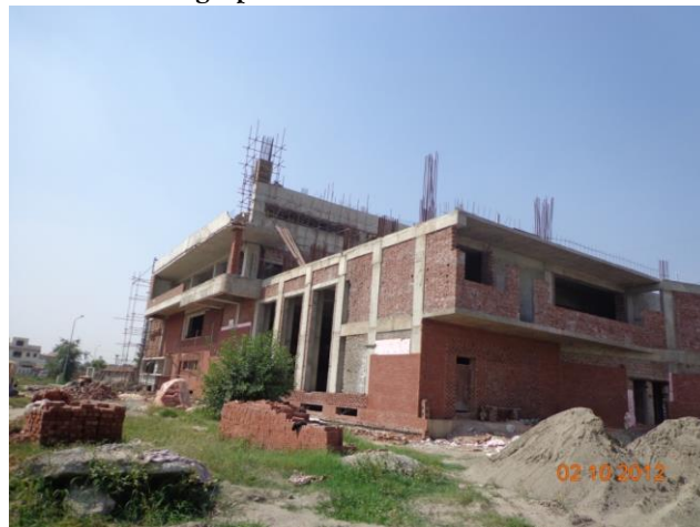
Fig 1 Building under construction rear view
